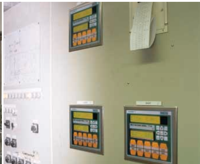
The systems T and Z provides computerized control of weighing. Rugged design and reliable performance makes them ideal for belt scale applications
